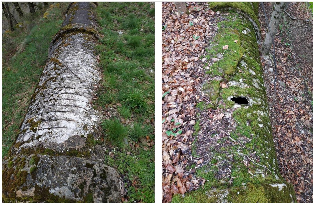
**PHOTOGRAPHIES DES DIVERSES DEGRADATIONS DE LA CONDUITE D'EAU FORCEE**
